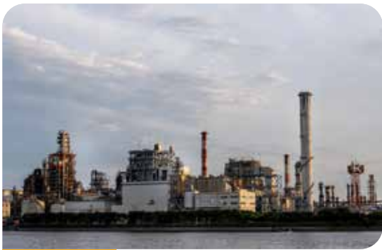
Primary & Secondary structures for boilers & turbine generators
