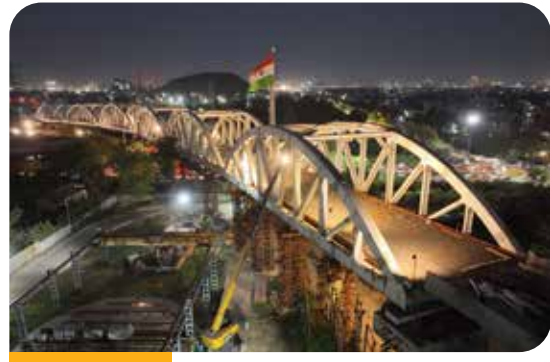
Structures for roads & bridges
